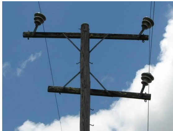
Figure 6 - 66 kV delta pin construction
