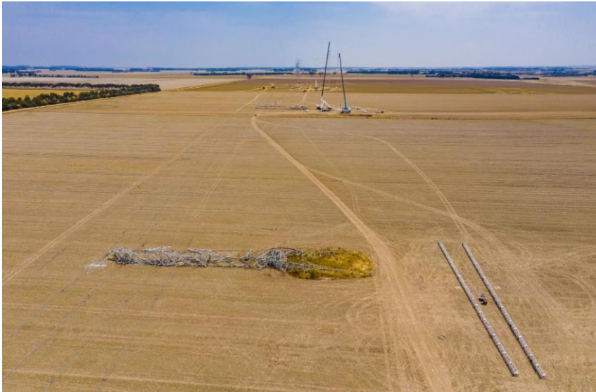
Figure 3 Damaged transmission towers
